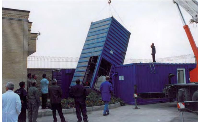
Erection of test systems on the grounds of the well pump station in Mashhad
