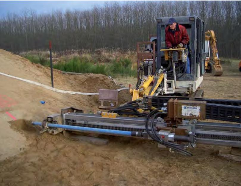
Standard drilling is to be applied to implement the linear drainage elements in the model dyke (Performed by: Morath GmbH, Albruck)
